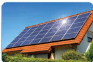
3 geothermal power/solar power
